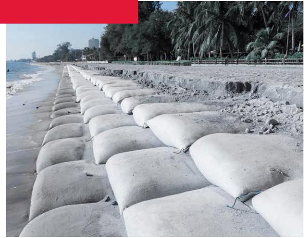
Preparing for a Hurricane page 06
